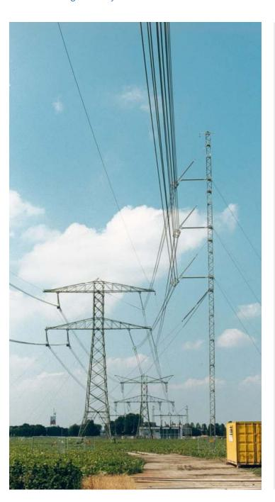
A tower of 30 metres high, using 10 mast sections, can be fully erected with the insulators in four hours: without a crane. The hoisting tower can be set up in areas where cranes or heavy vehicles cannot come.
